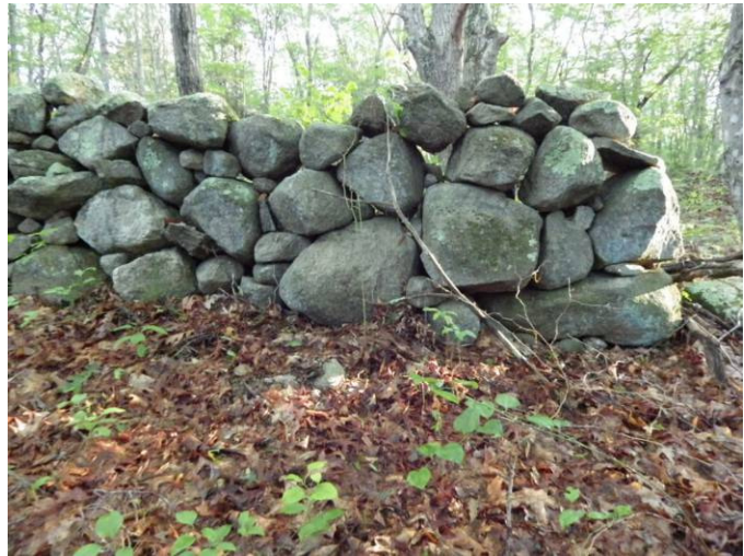
Opposite end has a finished end wall
