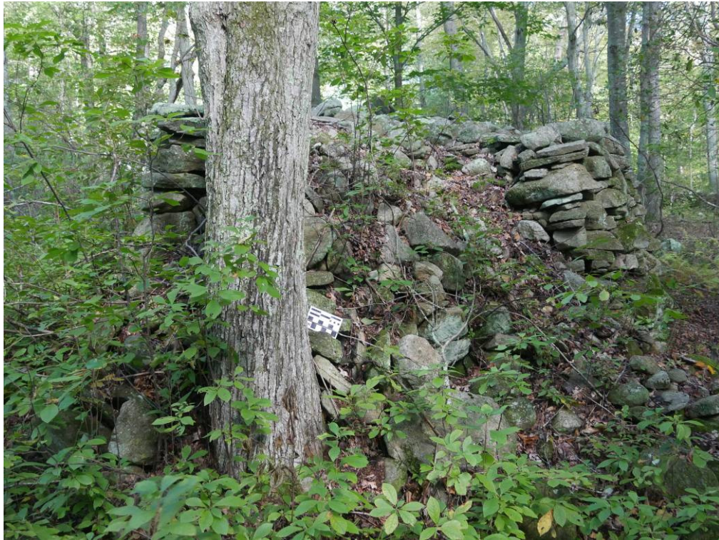
The end of the walls at the opening have a finished appearance indicating the opening is intentional rather than the result of collapse
