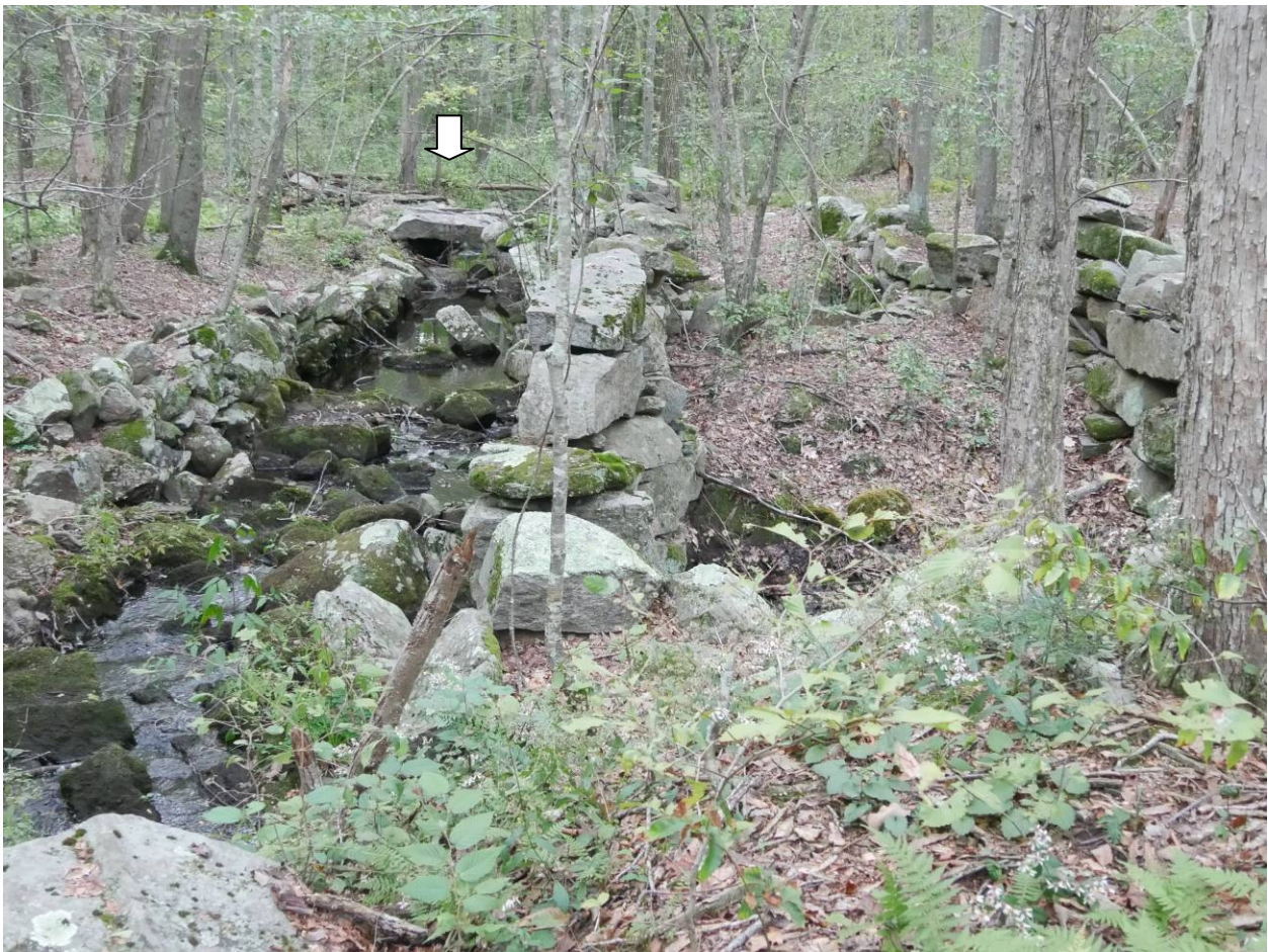
View of the sawmill foundation from the mill dam (looking south). Arrow points to a quarried stone culvert over the brook (downstream of mill foundation).
