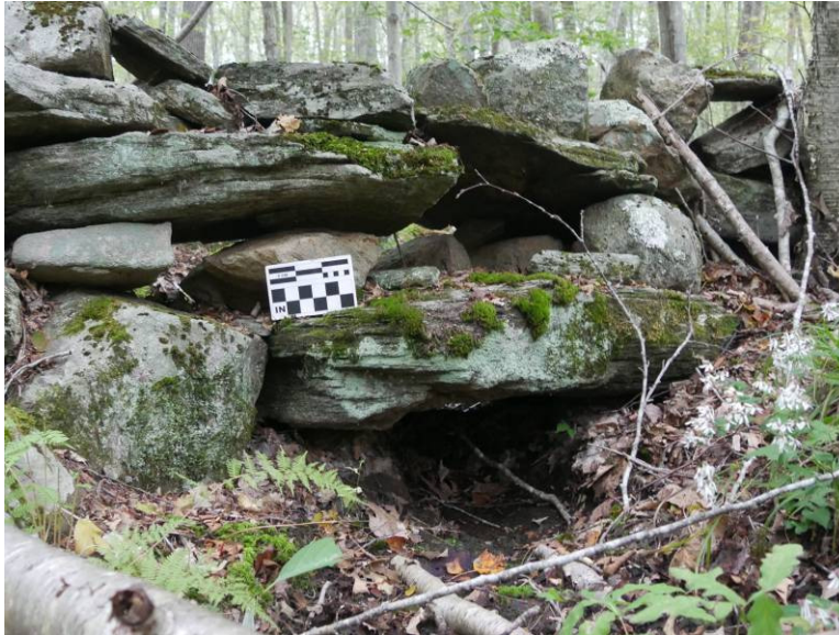
Culvert under stone wall adjacent to seasonal stream
