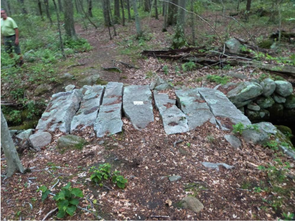
Culvert made from quarried stone bars built over Canonchet Brook
