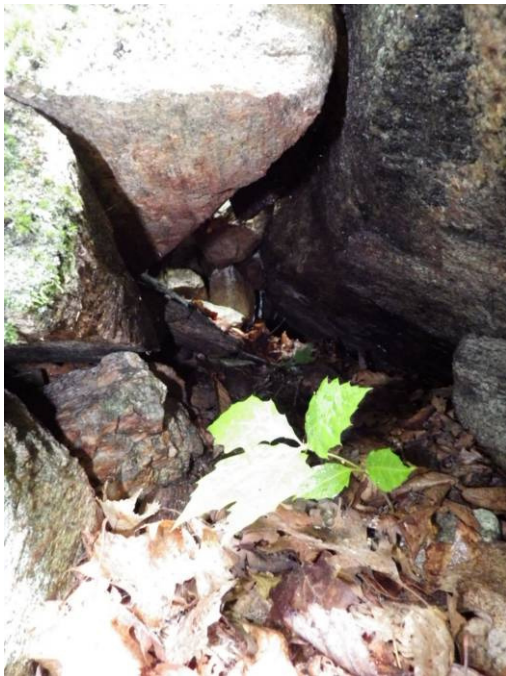
Interior of the open channel
