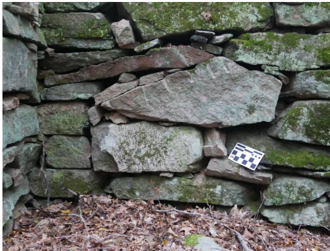
Quarried field boulder (Plug & Feather Method – 1820 or later)
