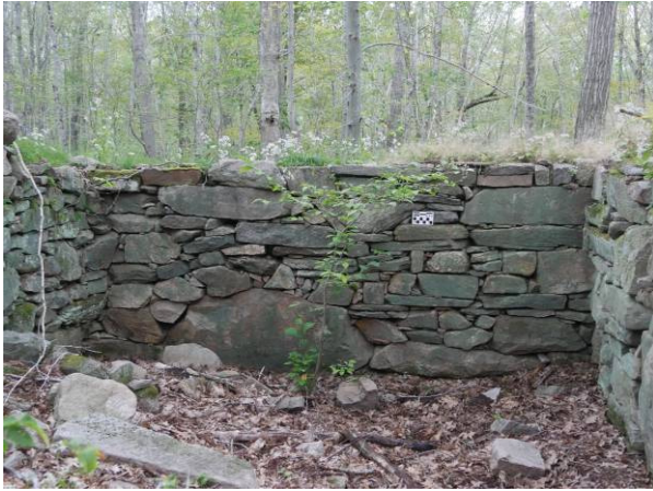
Interior view of cellar
