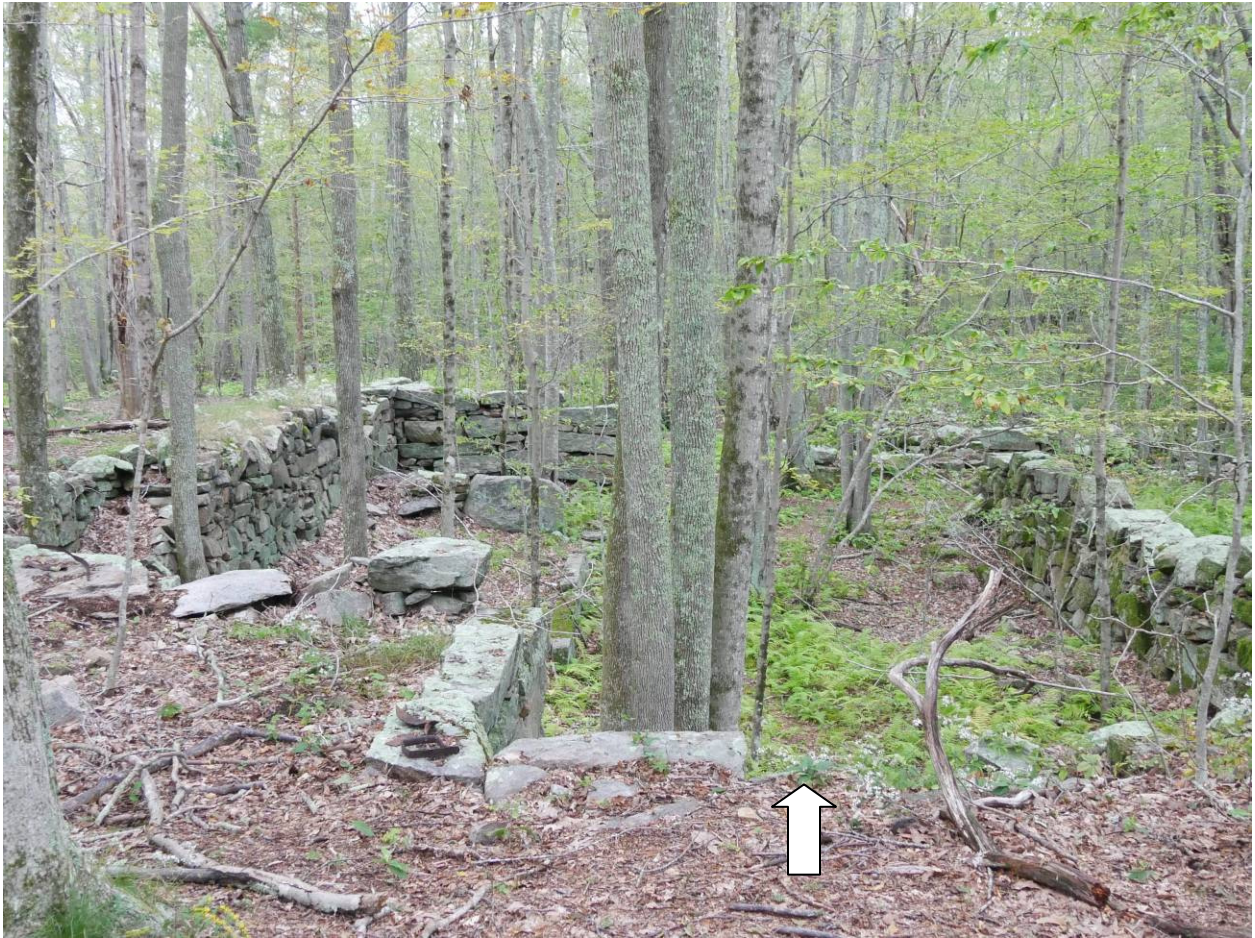
Overall view of the barn. Root cellar is in foreground (arrow).
