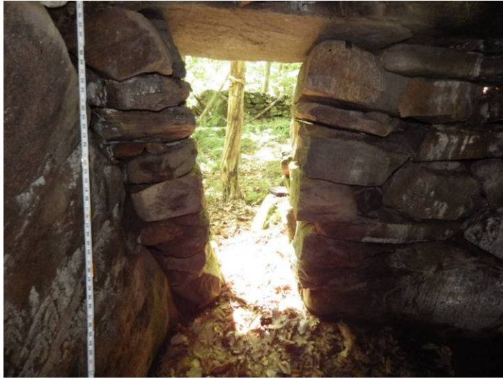
Looking out the entrance from inside
