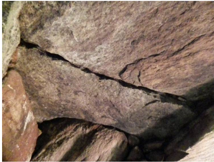
View of roof slabs
