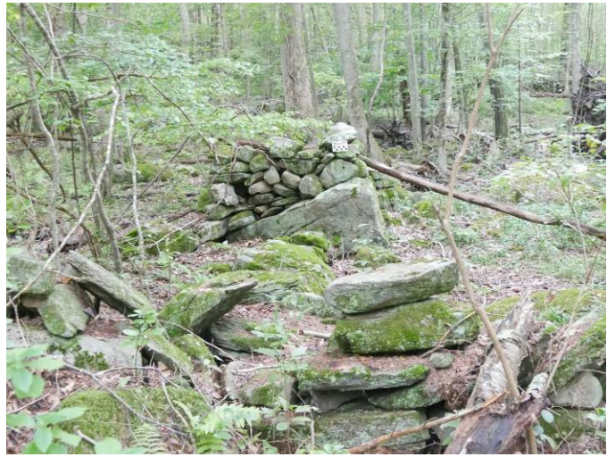
Wall in the foreground is the perimeter wall around the Center Area
