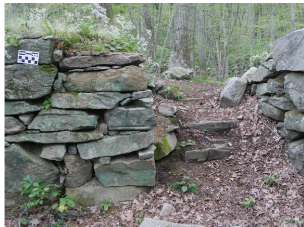
Exterior bulkhead stairway into cellar
