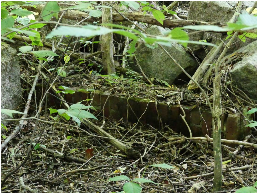
Figure 17 – Square brick column lying on its side.
