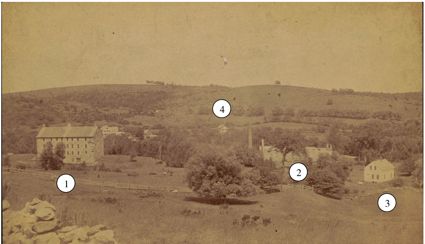
Figure 60 - Historic photograph (circa 1884-1896) showing a panoramic view looking to the north. (1) The stone boarding house (2) Fire damaged stone mill with large brick chimney to the left (3) The last of four wooden houses rented to mill employees, the other three having been demolished or removed from the property (4) Willowdale school house in Ipswich
