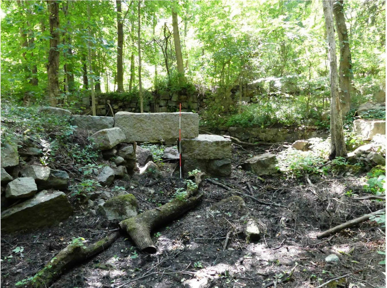
Figure 11 – Culvert in north wall of mill foundation that directed water out of the mill into the tail race. It is similar to sluiceway but on the water outlet side of mill. Funnels water through a stone lined channel back to river.
