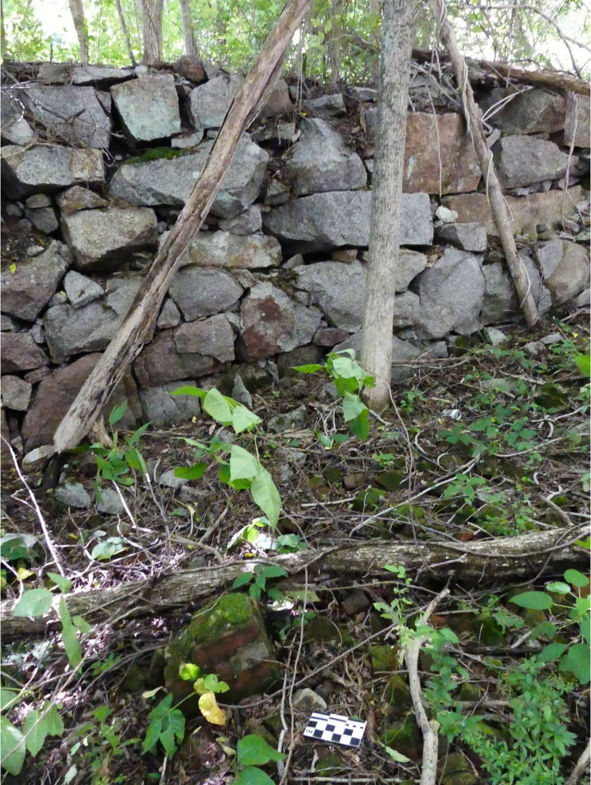
Figure 2 – South wall of mill foundation.
