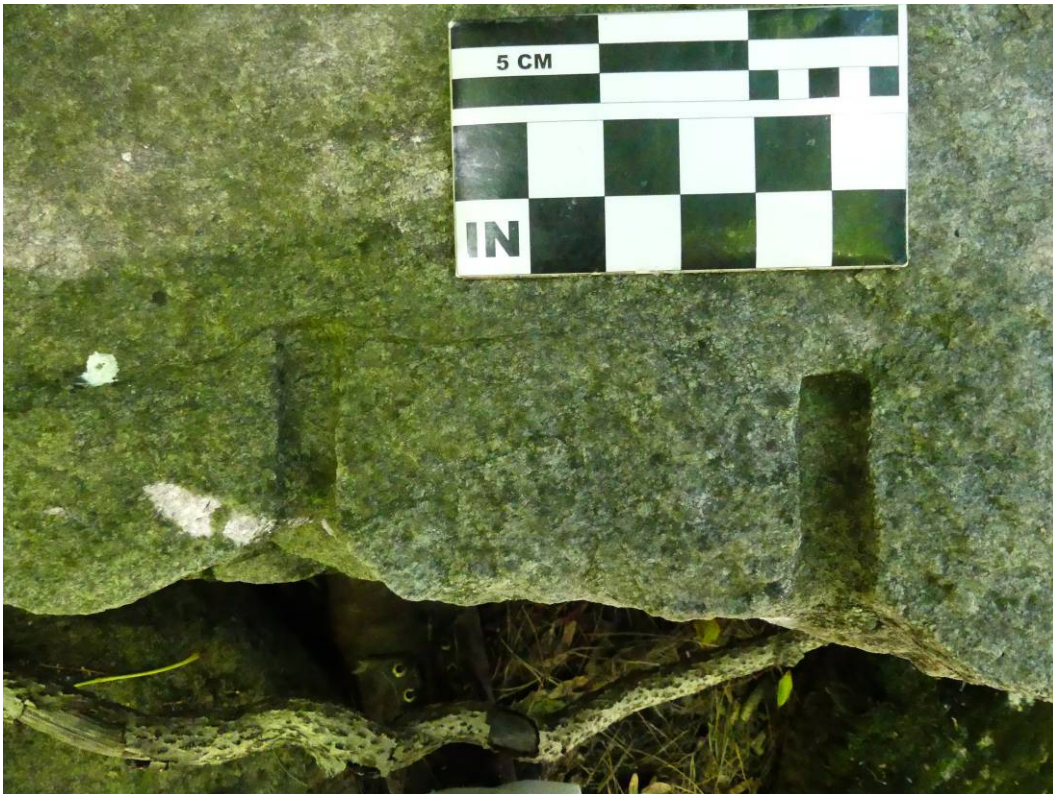
Figure 49 – Quarry marks from the plug 'n feather method.
