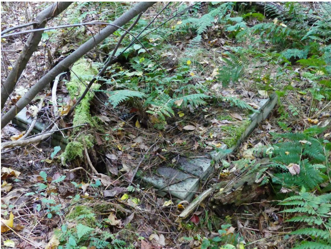
Figure 66 – Well covered for safety
