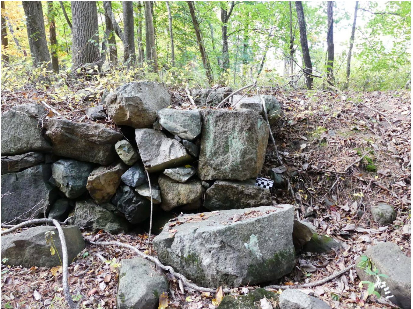
Figure 43 – The finished end wall of the sawmill foundation.
