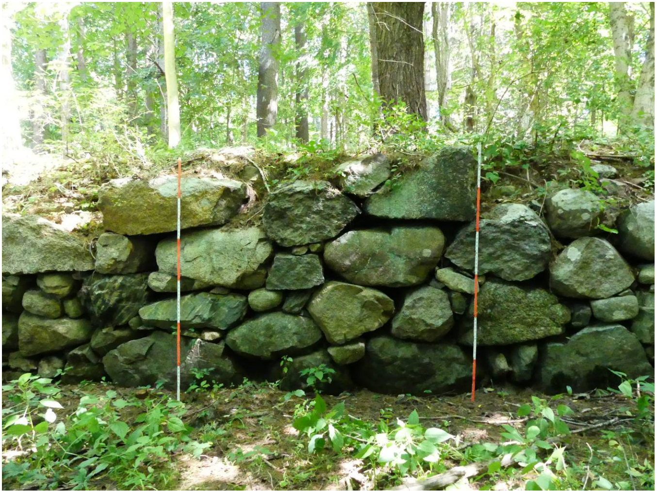
Figure 41 – The split boulders were augmented by and intermixed with unsplit boulders.
