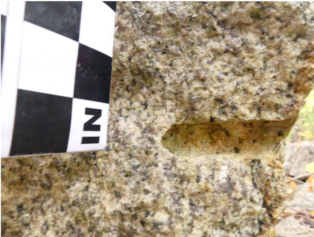
Figure 52 – The typical rounded bottom of a hole drilled with a plug drill.
