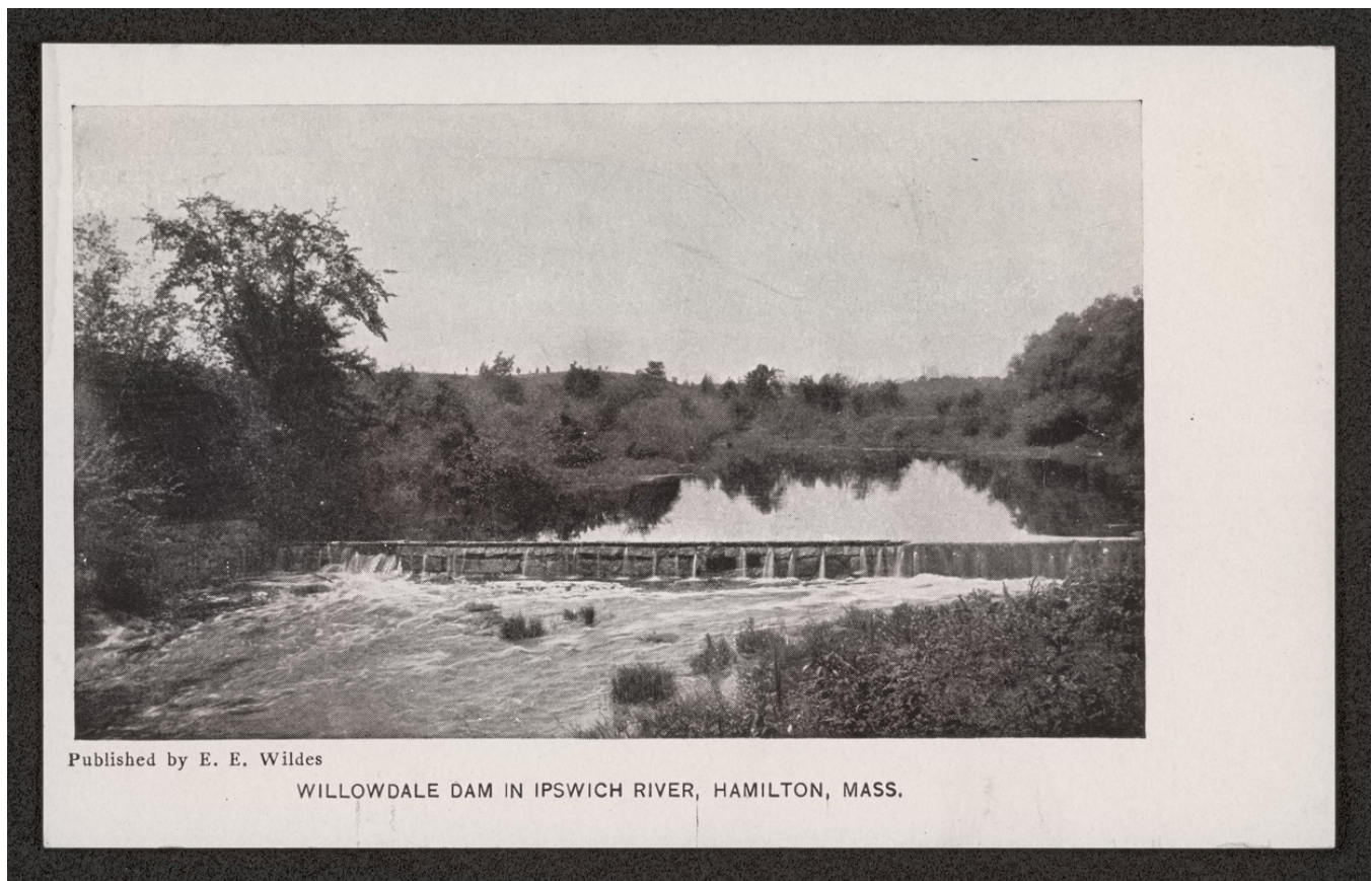
Figure 78 – Circa 1905 postcard view of the Manning / Willowdale stone dam Courtesy of the Hamilton Historical Society.
