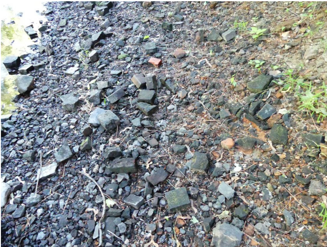
Figure 72 – Bricks and coal eroding form embankment of river.
