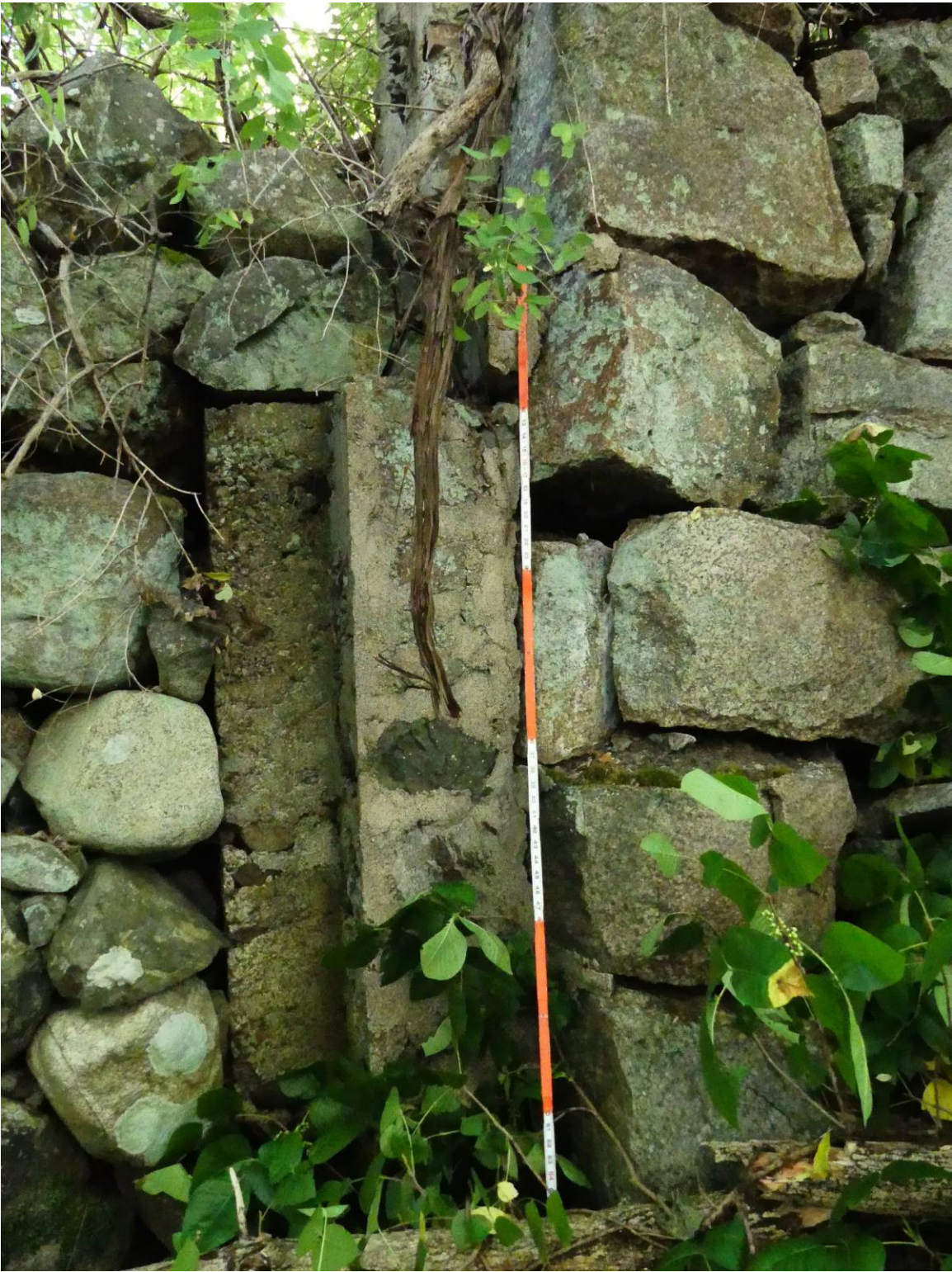
Figure 4 – Form pour cement wall on west side of intake opening.
