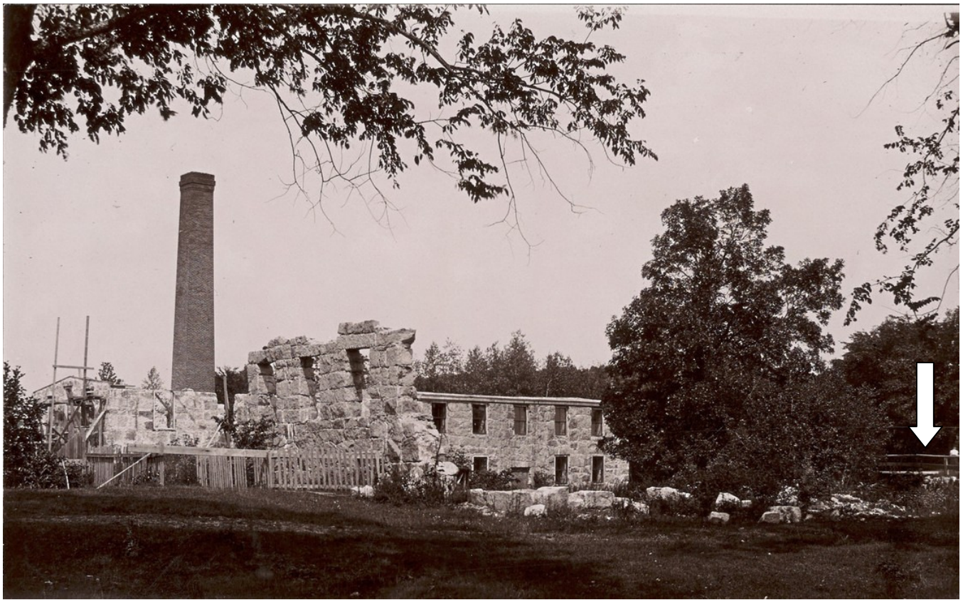
Figure 37 – Historic photograph (circa 1884-1896). This photo was taken at a similar angle to the one of figure 36. Over 90% of the upper story stonework of the mill have been dismantled and removed. It is unclear from this photo how much of the foundation stonework was dismantled by this point. The stone ell is visible in the background. Part of its roof was damaged during the fire and is missing on the far left of this photo. On the right side the roof is intact and windows are still in place. The bridge over the tail race and Ipswich River is just visible on the right edge (indicated by the railings – arrow points to it.)
