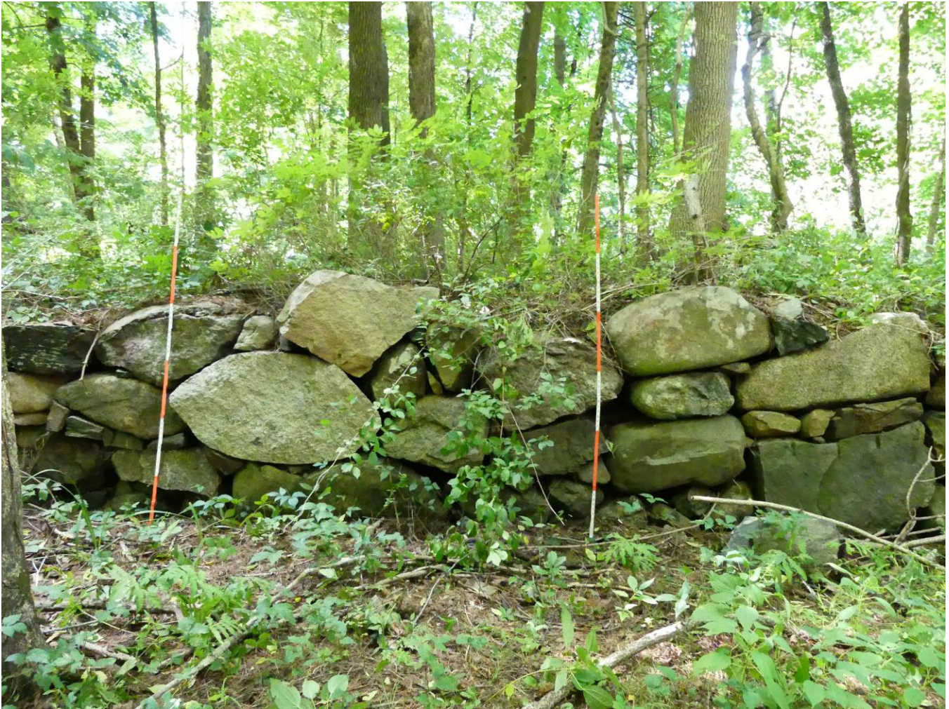
Figure 39A – The veneer sawmill foundation was constructed of a mix of unsplit and split field boulders.
