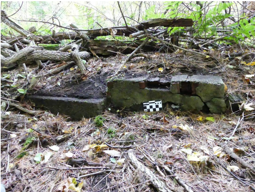
Figure 64 – Low foundation sill wall with cement covered bricks and a possible doorstep on far left end.
