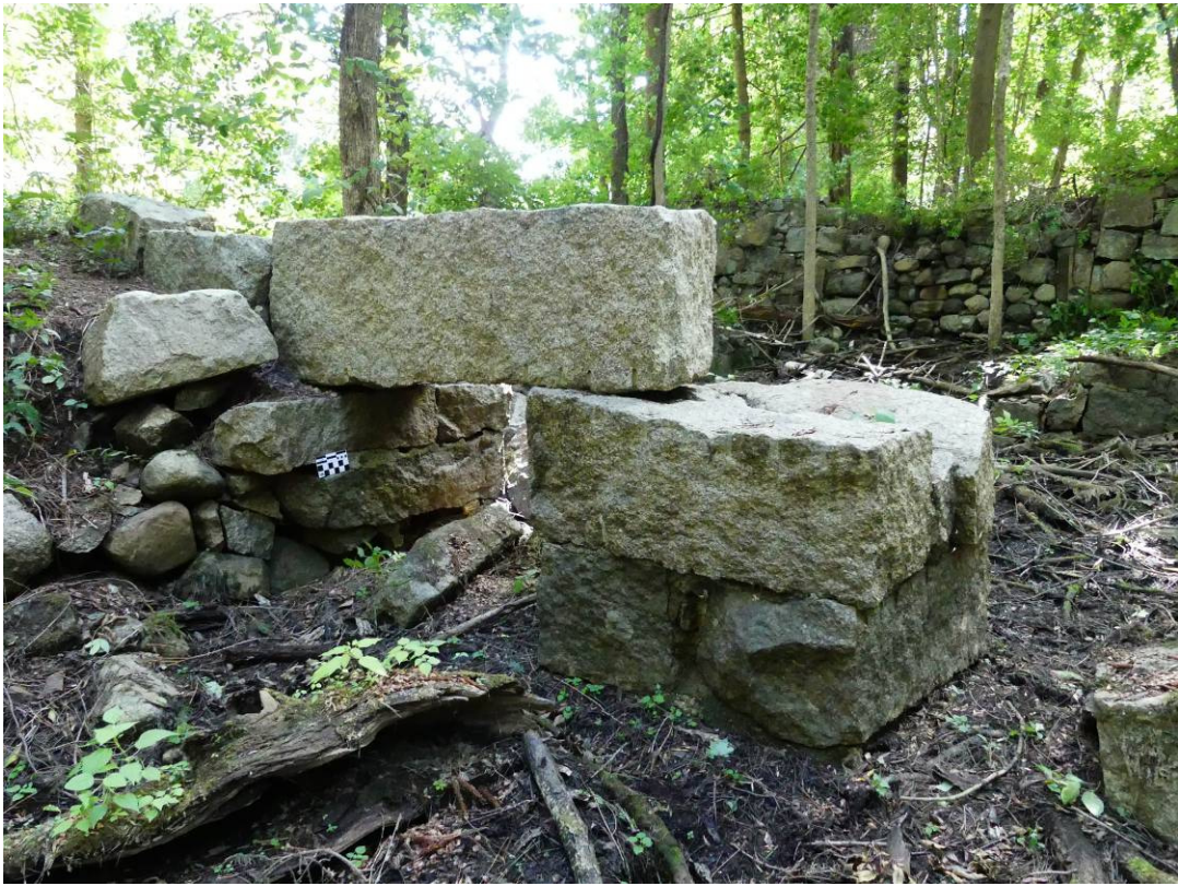
Figure 12 – Culvert was constructed of large blocks of quarried stone.
