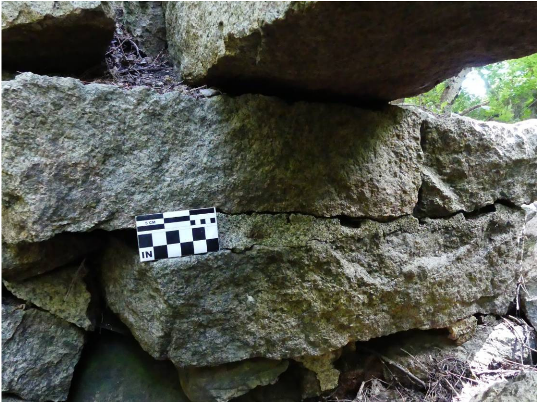
Figure 13 – A small amount of mortar was used.
