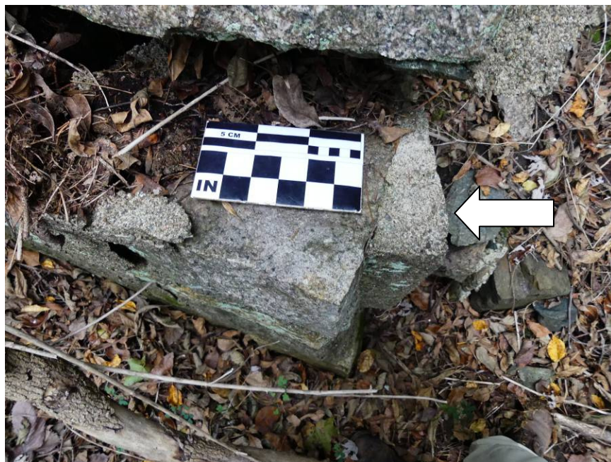
Figure 32 – Top down view of form poured cement feature with slot for wooden vertical beam.
