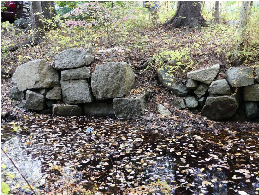
Figure 26 – A section of intact walling along tailrace.
