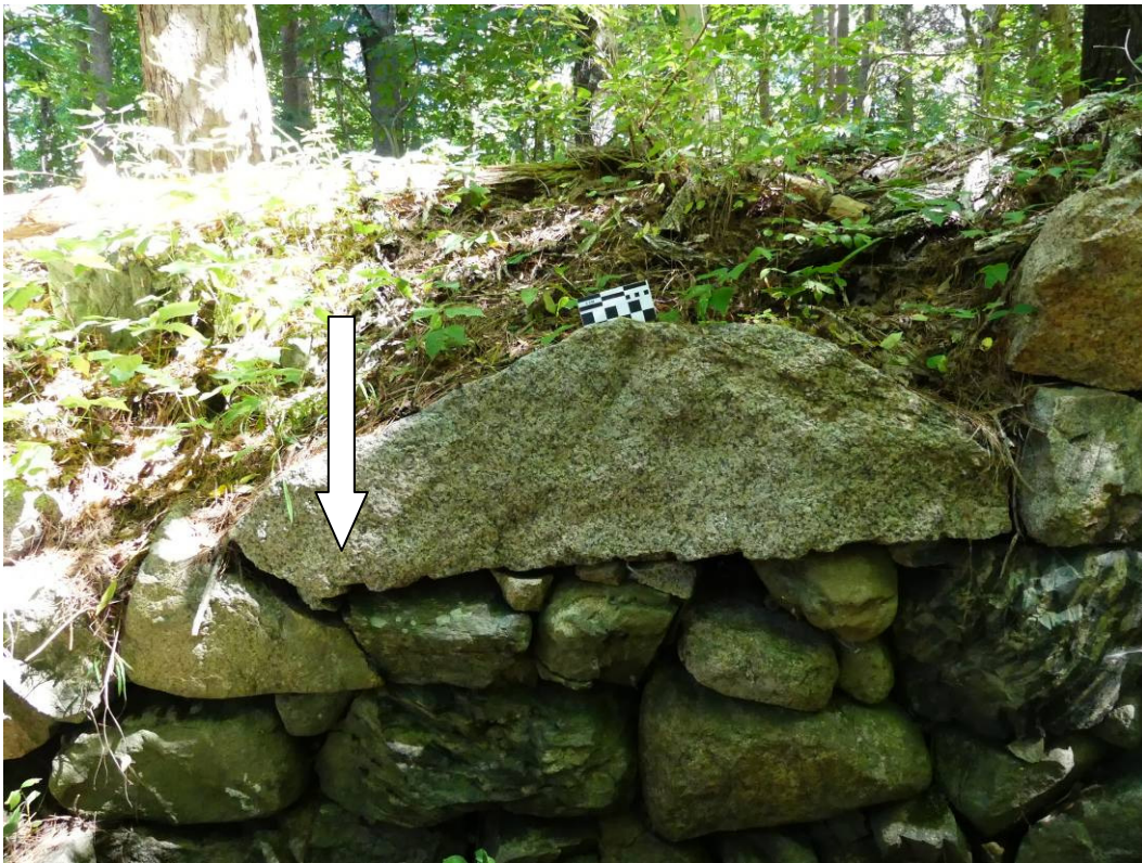
Figure 46 – A single hand chiseled flat wedge quarry mark was found mixed in with half round drill holes.
