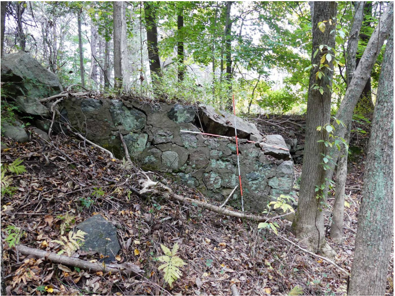
Figure 30 – Angled stone and cement wall. (View from inside canal)
