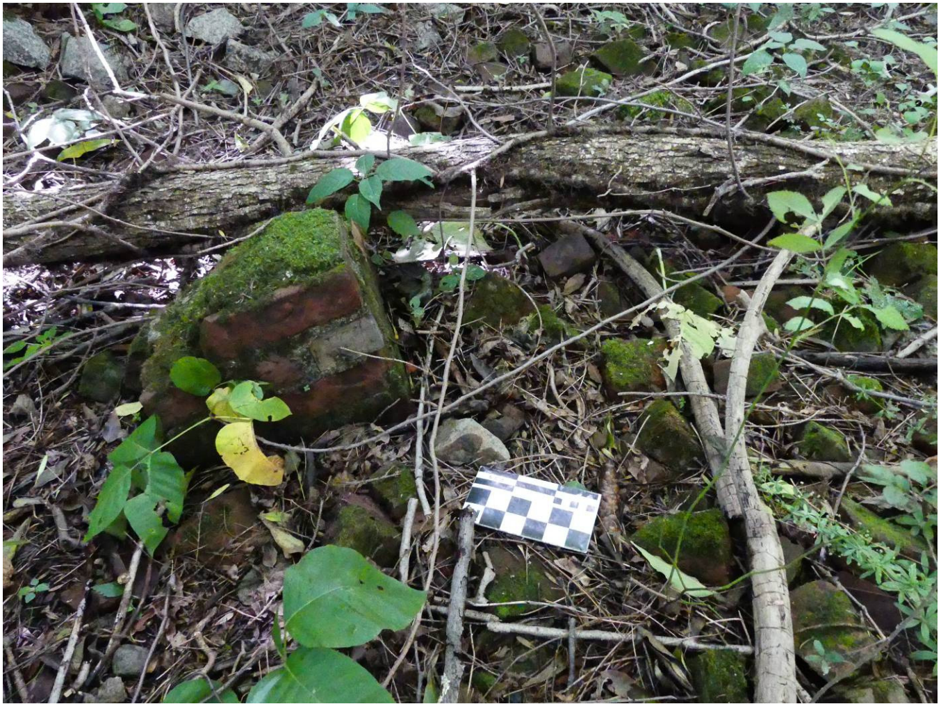
Figure 15 – Wide pile of loose bricks was located adjacent to the south wall west of the intake opening. Among the loose bricks are several segments of cemented bricks.
