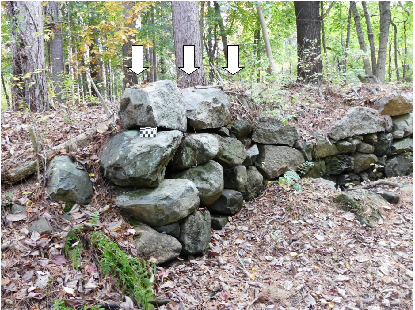
Figure 44 – Rebuilt section of the tail race just after the end of the sawmill foundation. It curves inward. It located opposite of the foundation end wall shown in fig. 43. Arrows indicate rebuilt section.
