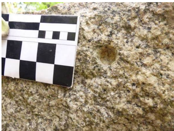
Figure 23 – “Dog hole” – Shallow hole used with large hooks and chain to lift blocks. The hooks fit into the shallow holes so they grip the block.
