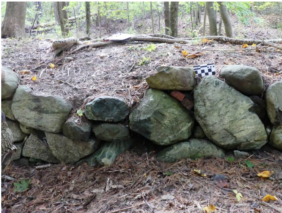
Figure 58 – another view of the retaining wall.
