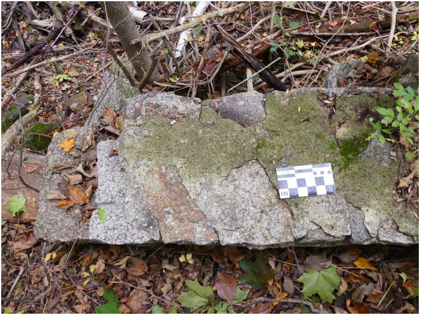
Figure 18 – Top of south and west wall had a thin layer of cement.
