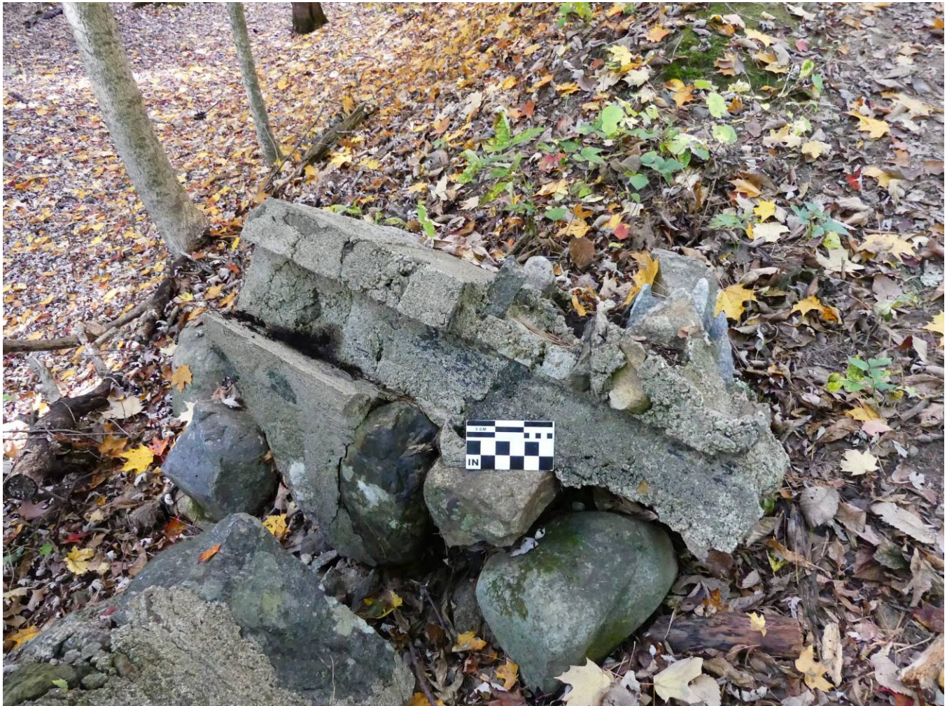
Figure 55 – Remains of one of the form poured cement abutments at the opening between the canal and sawmill foundation. It dates from Francis Dane’s ownership of the property (1897-1902). It was used for a control gate. According to life long local resident Bob Foote, the slot was in upright position and formed a stop log (i.e. boards placed inside slot) gate to control the water. The abutments were damaged and knocked over in the Mother’s Day flood of 2006.
