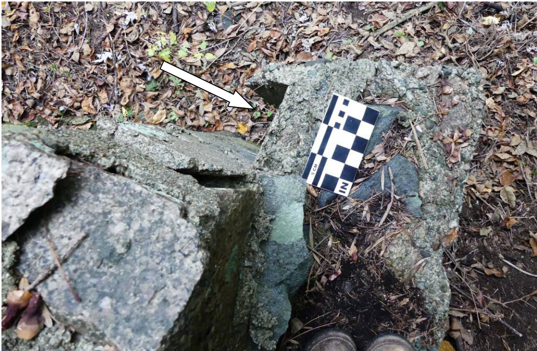
Figures 29 – Form poured cement feature with slot for vertical wooden beam.
