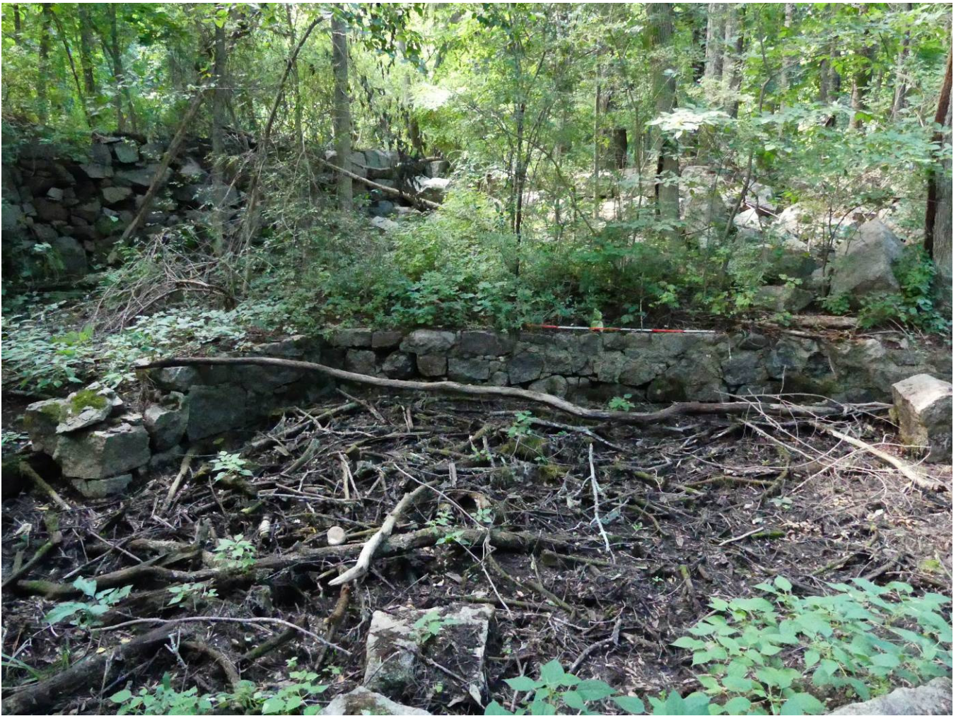
Figure 7 – 2 nd Low stone & mortared wall with an L shape extends from about the center of the interior out to north wall of the foundation next to a culvert, water outlet feature.
