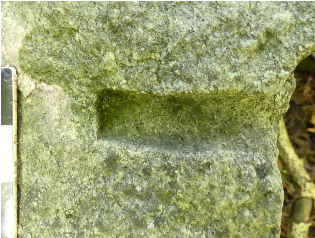
Figure 50 – These holes are highly usual because the bottoms are flat rather than the rounded.
