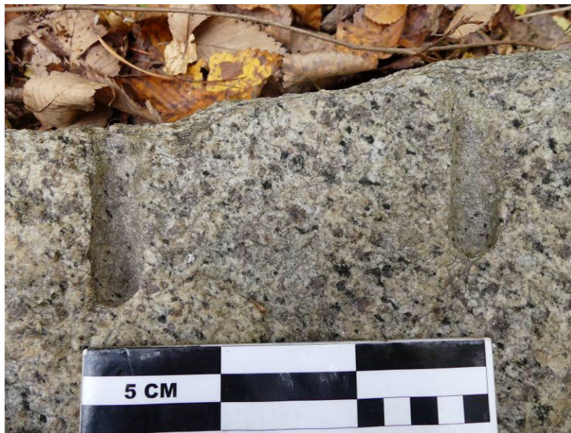
Figure 21 – Close-up of half round drill holes from plug and feather method.
