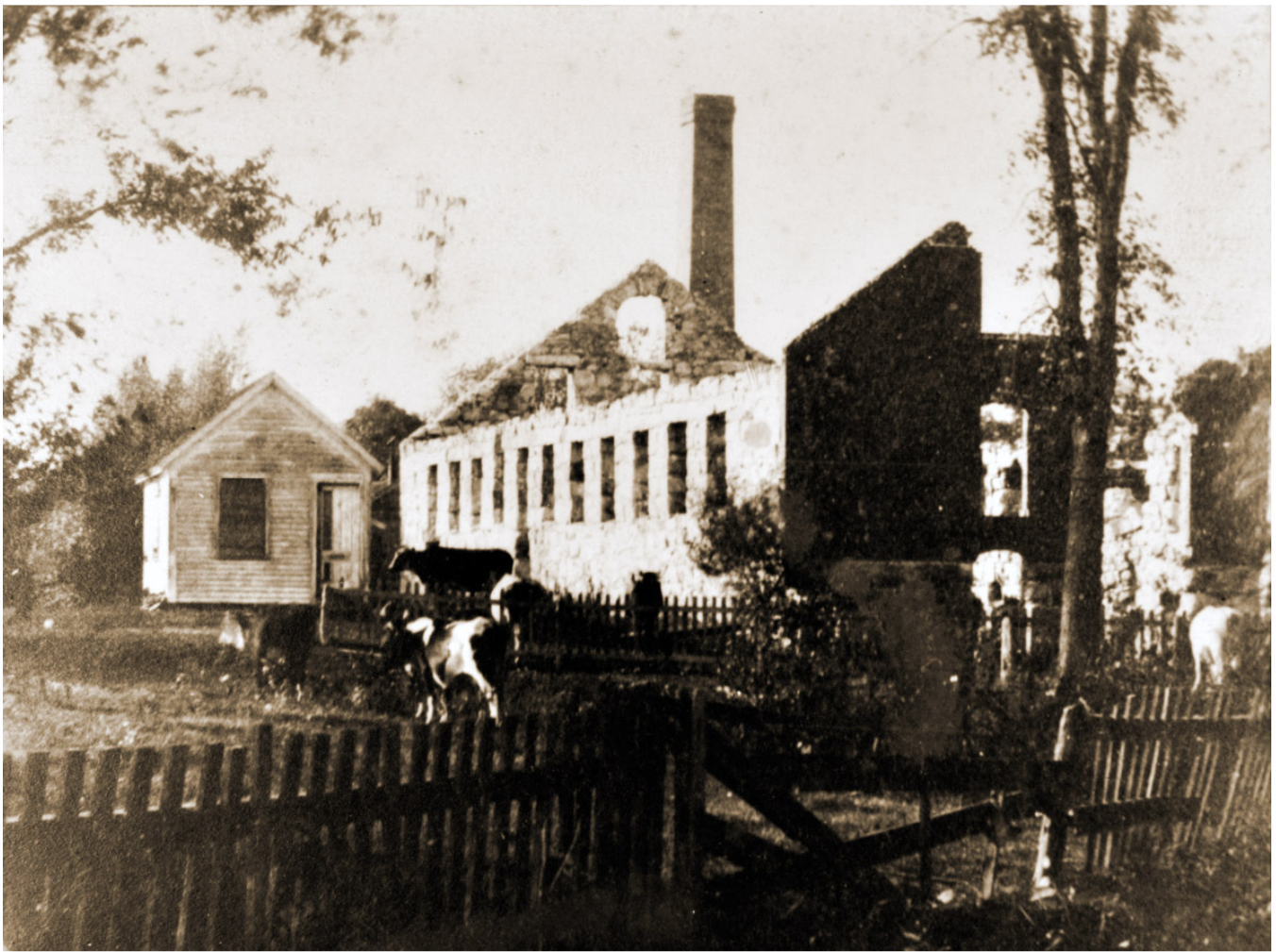
Figure 36 - Historic photograph (circa 1884-1896) of the fire damaged stone mill (looking northwesterly). The photographer was standing near or on Winthrop Street. The wooden building at the end of the canal is shown and a door is visible on this side. Cows are grazing. This photo shows details of the end walls of the mill. The far (west) end wall was stone and an opening for a large window is present. About 2/3rds of the front façade end wall (which faced the road) was still standing. This wall was identified as being made of brick in the photo in figure 35. The front wall has a single window at the bottom with a window directly above it, another above that one, arranged vertically. This is a small but critical detail when compared to the window configuration shown in fig. 38)
